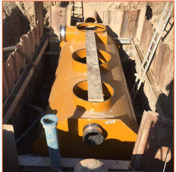
Factory Rastatt– GERMANY Treatment plan 30 l/s
